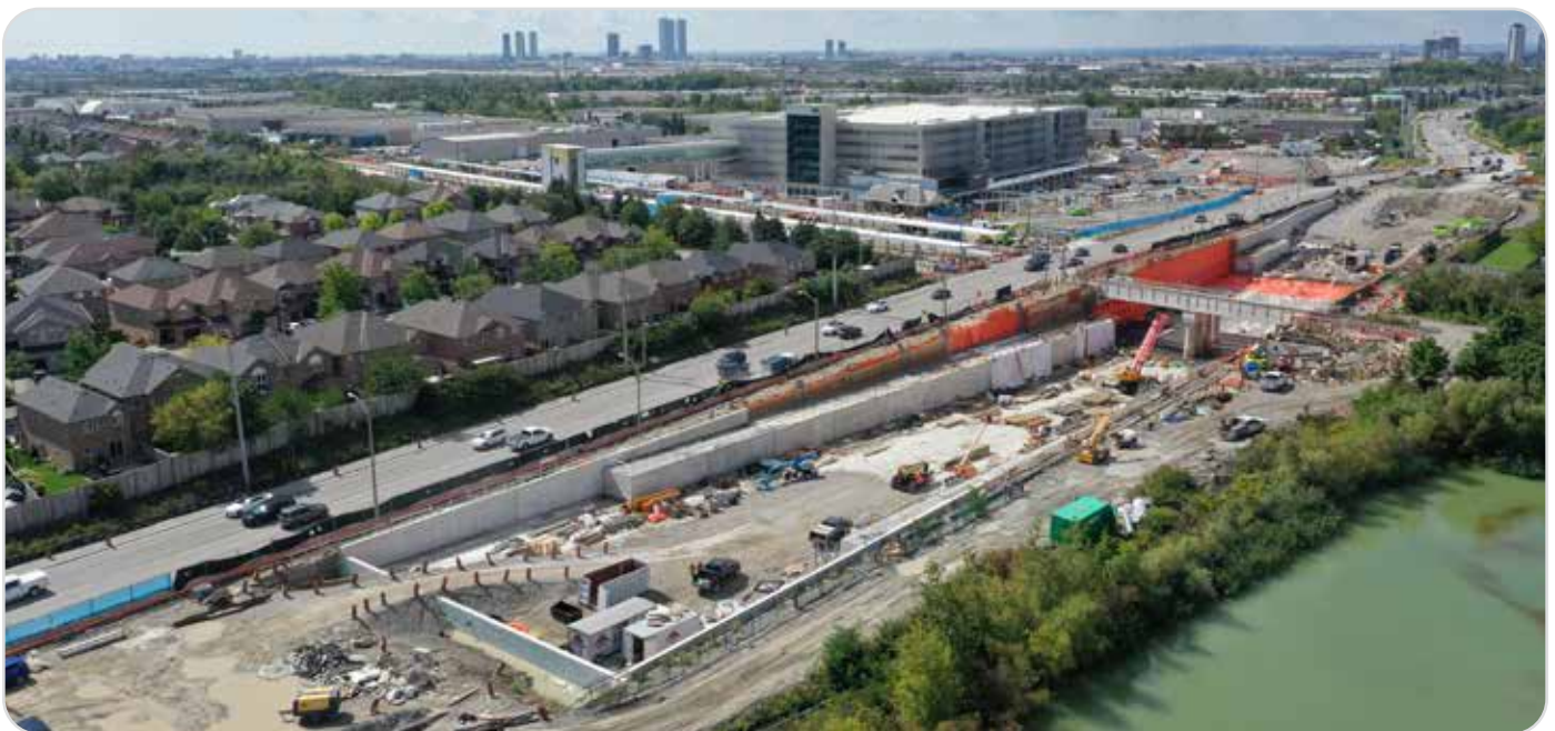
▲ Construction of Rutherford GO rail grade separation on Rutherford Road in the City of Vaughan.
