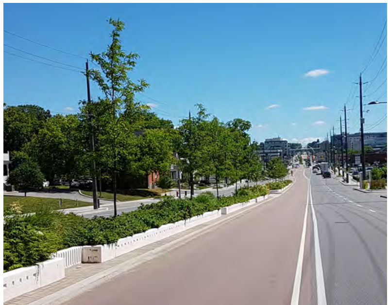
Raised concrete planters along Viva Rapidway
