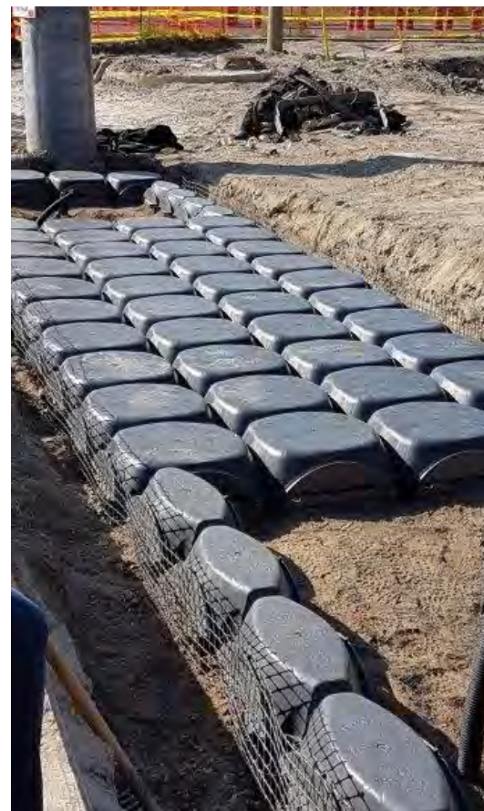
Installation of a soil cell system
