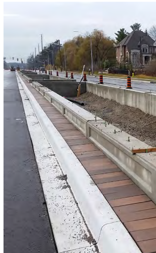
Raised median before installation of Region designed soil
