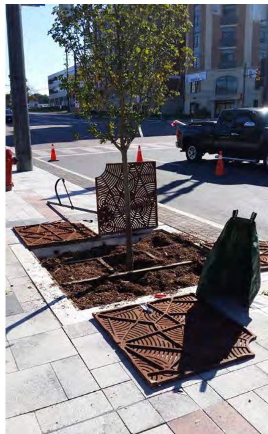
Tree grate installation
