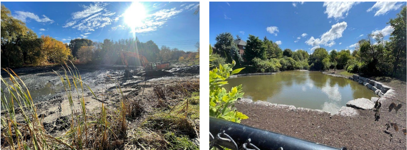
Figure 2: Pond 44 during cleanout (left) and Pond 73 after cleanout (right)
