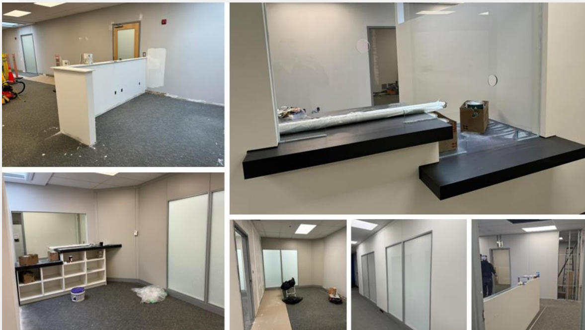
Figure 2. Newmarket Processing Center Renovations.
