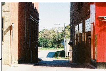
4: View looking east at lane between 197 and 201 Main Street South
