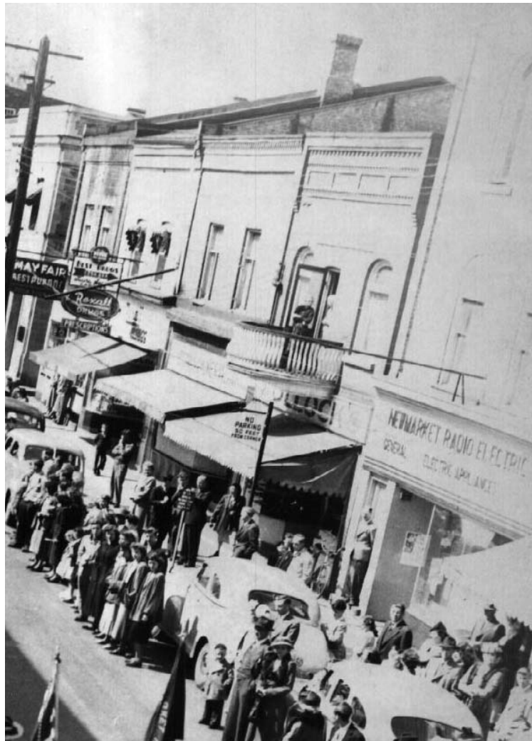
The historic photograph (digital photo 9865611 in the collections of the Newmarket Historical Society) shows the original central door in the upper storey of 223 Main Street South and a balcony which explains the bricked-in opening on the upper floor.
