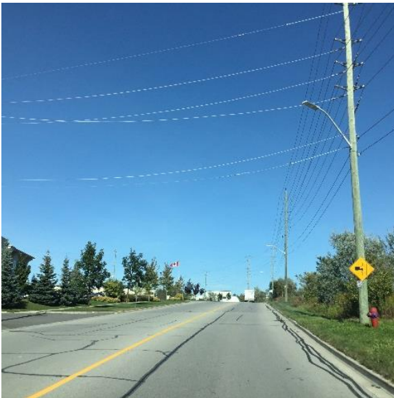
Existing Two-lane Road on Harry Walker Pkwy. Proposed to be a Buffered Bike Lane route
