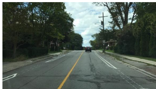
Buffered Bike Lanes on Srigley Rd. (East-West Bikeway)
