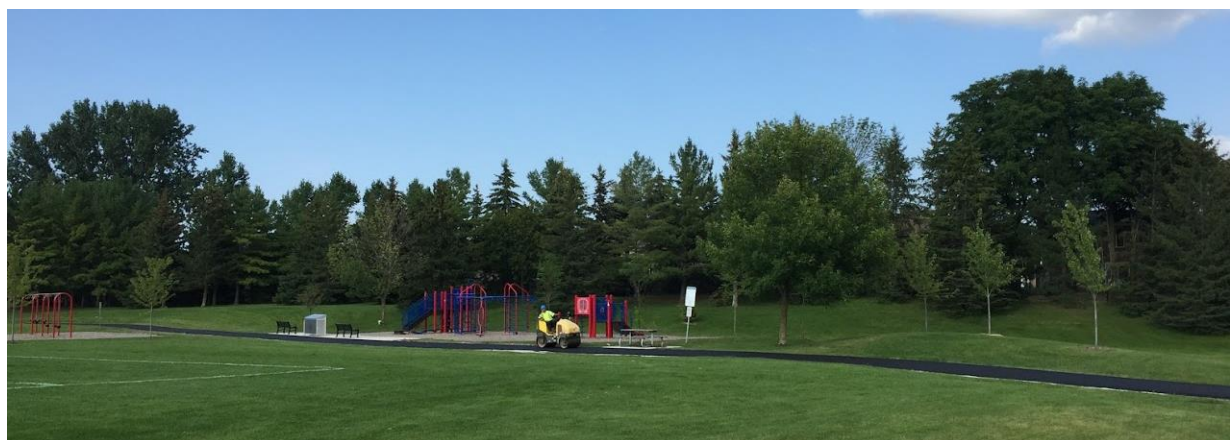
Trail maintenance and Re-surfacing at Joe Persechini Park
