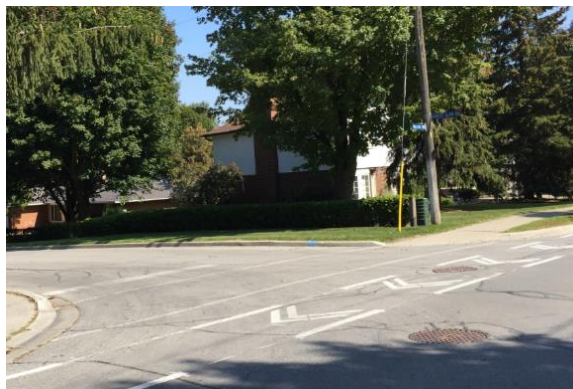
Bike Lane Crossing Markings (Chevrons and Skip Lines) in Newmarket on Millard Ave.
